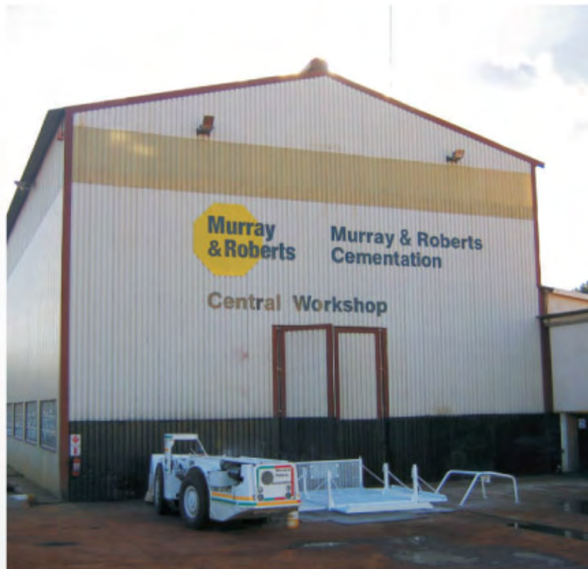
Bentley Park comprises a plant store yard, in-house workshop and training facility at its operations
