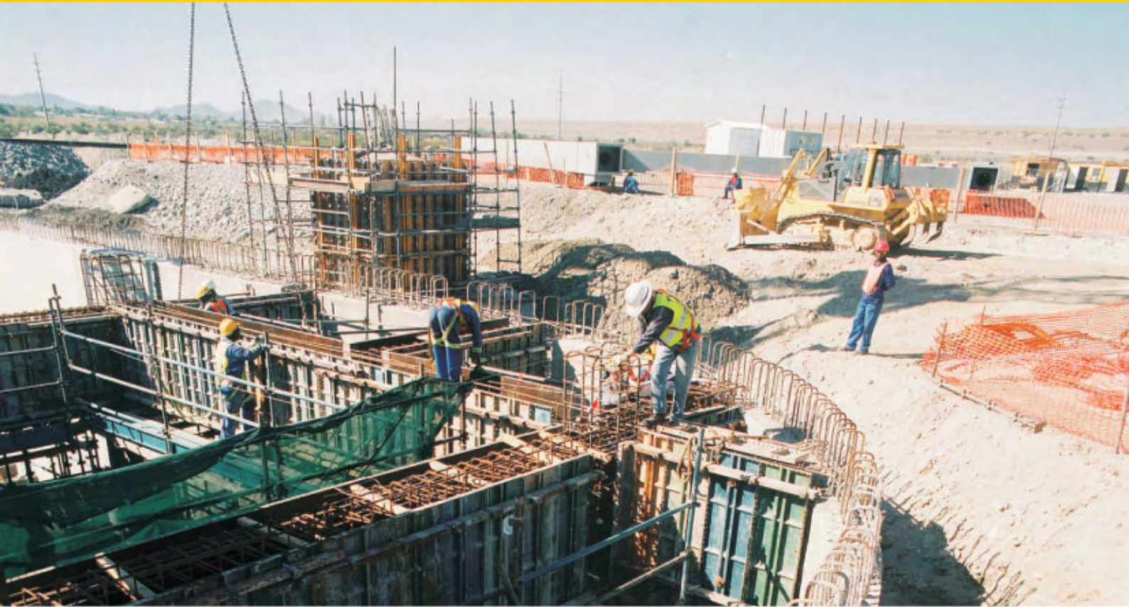
Construction of the collar
